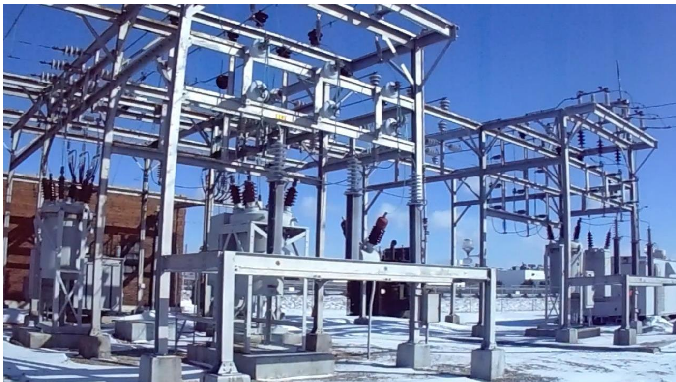
Photograph 2 – Yard Structure Arrangement
