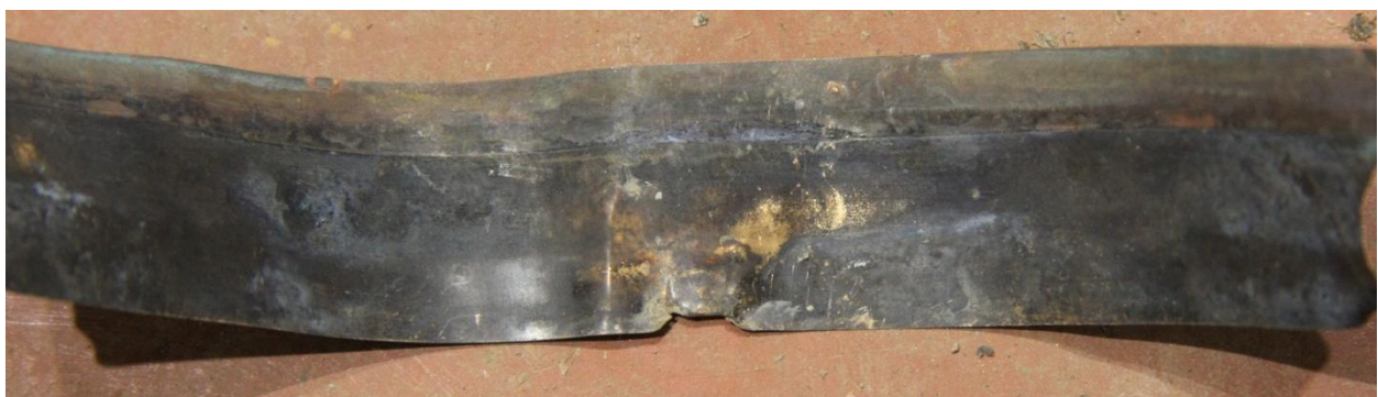
Figure 11: Possible Electrical Damage to the Metallic Tape Neutral
