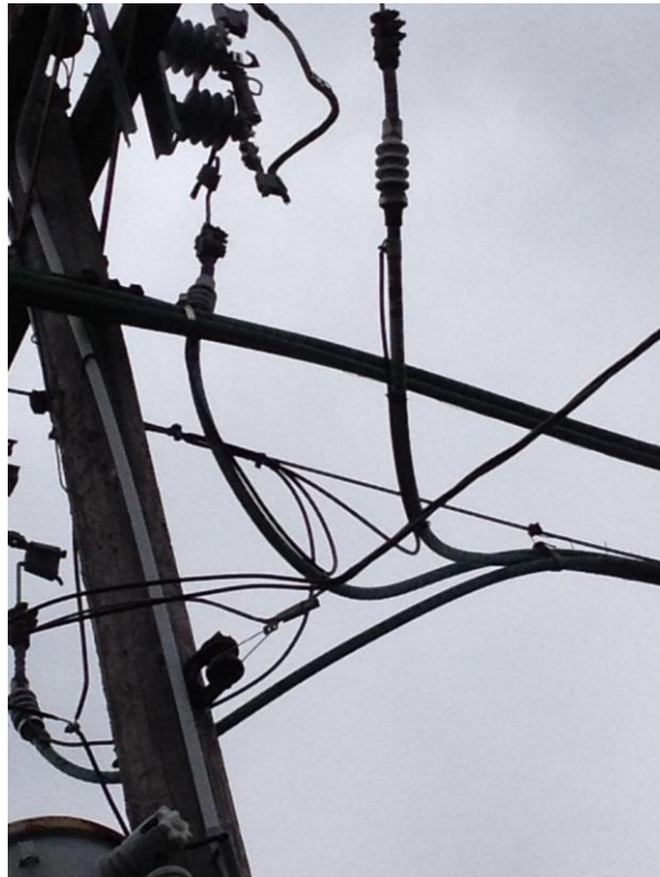
Figure 2: Cable as it was installed
