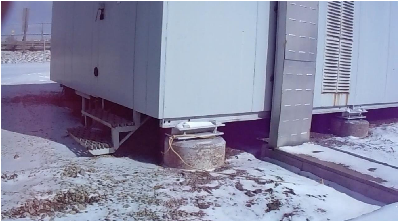
Photograph 10 – Switchgear Building Foundation
