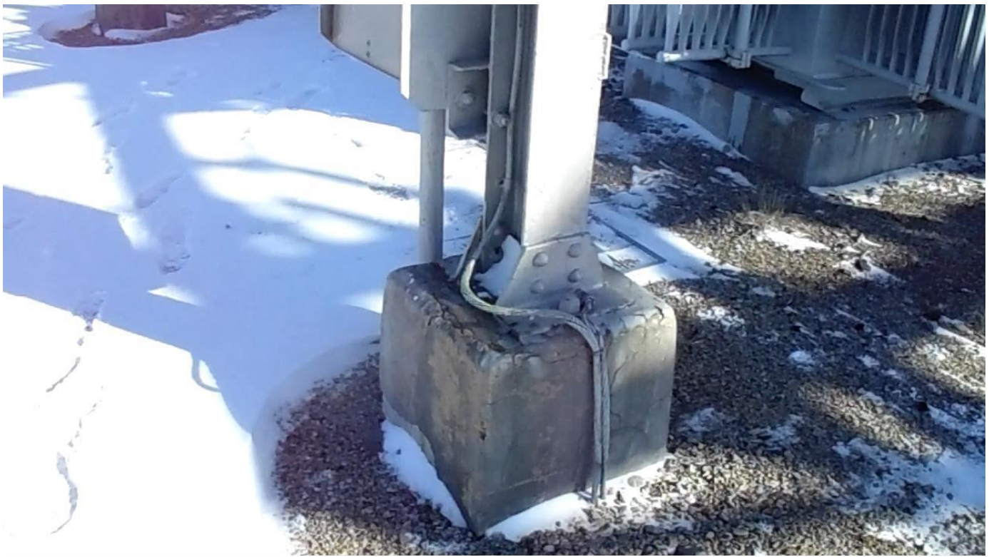
Photograph 7 – Repaired Concrete Pier
