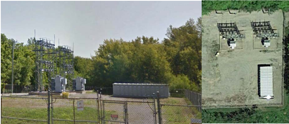
Figure 5.4.6.13-2: Street and Overhead View of Station 19 DS
