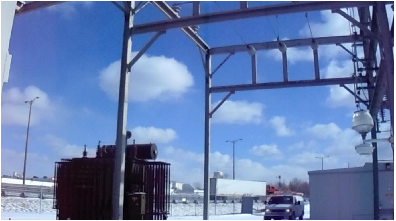
Photograph 5 – Knee Braces on Columns
