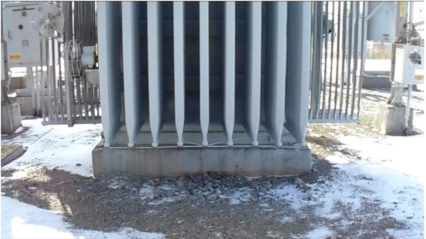
Photograph 9 – Bank #1 Transformer Foundation
